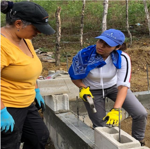
The 1 st poured concrete column within the wood form & laying the first blocks on it after the wood mold is pulled away.
