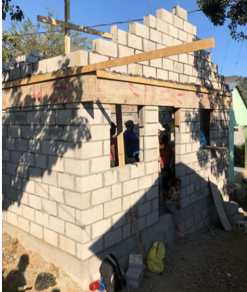
Triangular peaks on top of final horizontal poured beam
