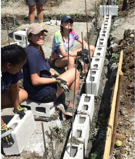
The 1 st poured concrete column within the wood form & laying the first blocks on it after the wood mold is pulled away.
