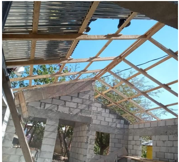
Wood forms in place on triangular peak to pour concrete to level the block & the wooden support rafters in place for the roof
