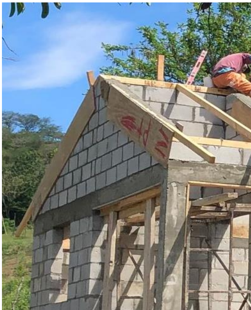
Wood forms in place on triangular peak to pour concrete to level the block & the wooden support rafters in place for the roof
