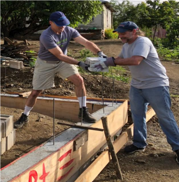
The 1 st poured concrete column within the wood form & laying the first blocks on it after the wood mold is pulled away.
