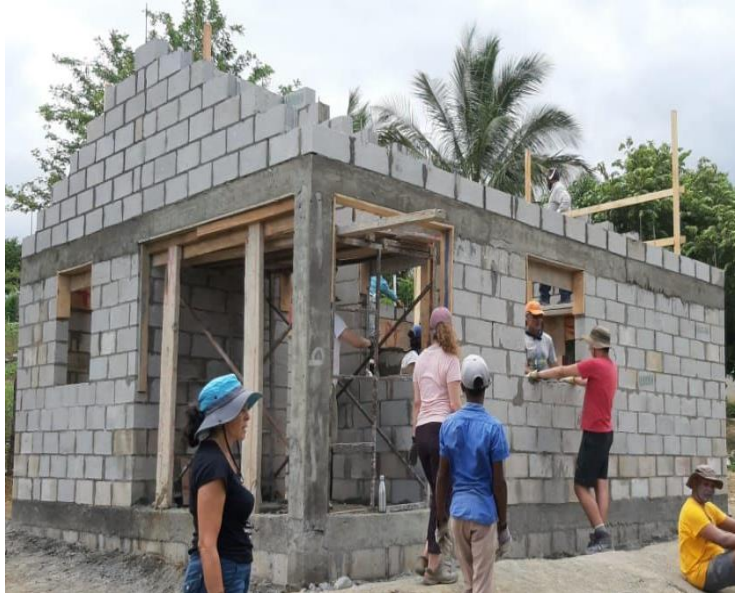
Triangular peaks on top of final horizontal poured beam
